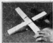
How does one rubber band hold a wing to a motor stick? This photo shows you.
