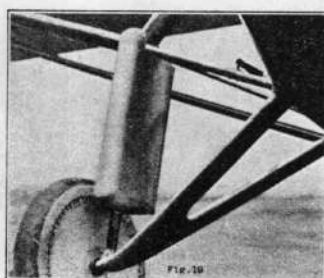
Note the smooth, streamlined struts.
