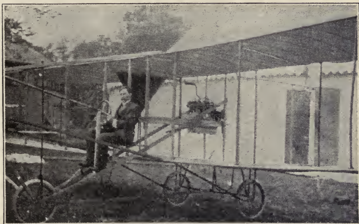
Position of Motor on Brauner-Smith Machine.
