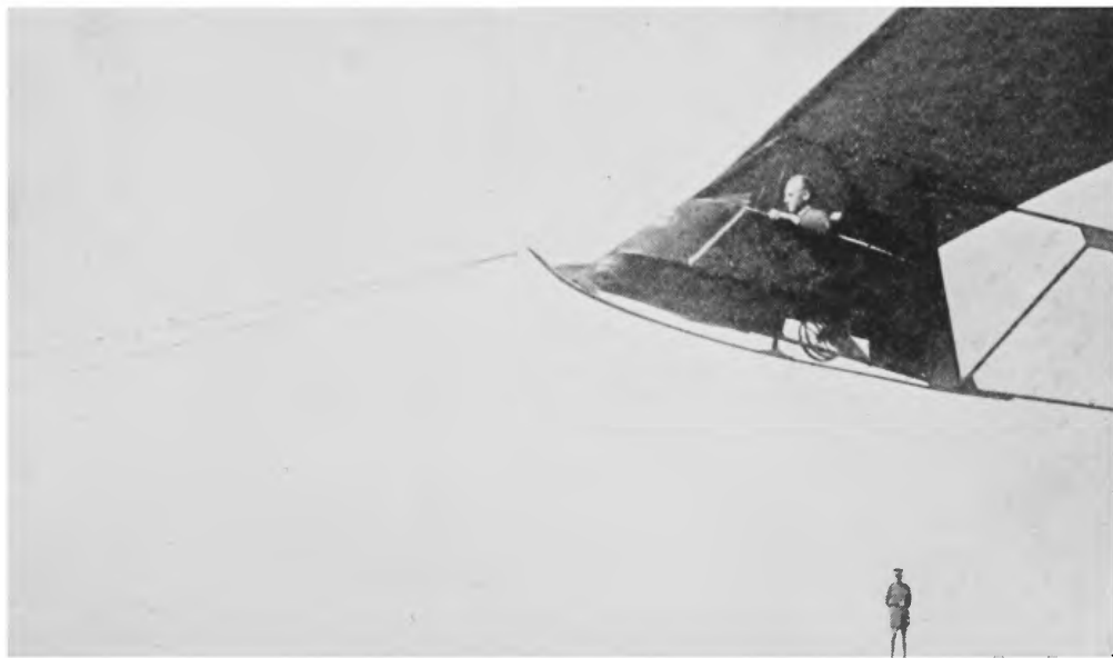
FIG. 42.—A glider with skid and auxiliary wheels. This skid absorbs the shock of landing. The wheels do not add greatly to the parasite resistance, since they are set into the fuselage.
