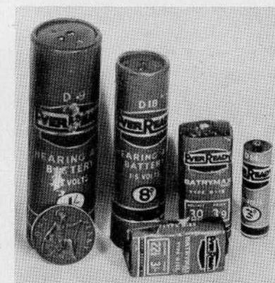
Average types of dry cells and batteries used for R.C. receivers. These are all "Deaf Aid" types, and are stocked by model and radio dealers all over the country.
