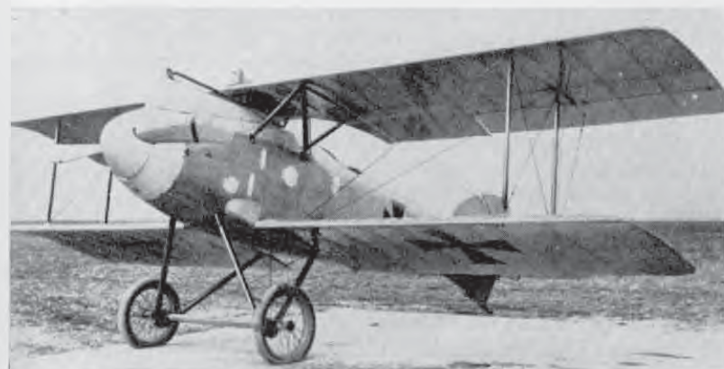
Albatros D II (Austrian-built, with centre-section radiator and Austro-Daimler engine). (Photo: Imp. War Museum.)
