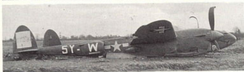
Right: P-38J, 364th Fighter Group, 385th Fighter Squadron, note flak damaged port spinner, Code 5E-H, serial painted out, white triangle on fin and rudder. (Ray E. Bowers)
