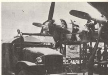
Men at work: B-29 ground crew probe the innards of a Superfort's starboard engines while a refuelling crew top up the tanks. The vehicle in the foreground is the ubiquitous GMC 2½-ton tanker.
