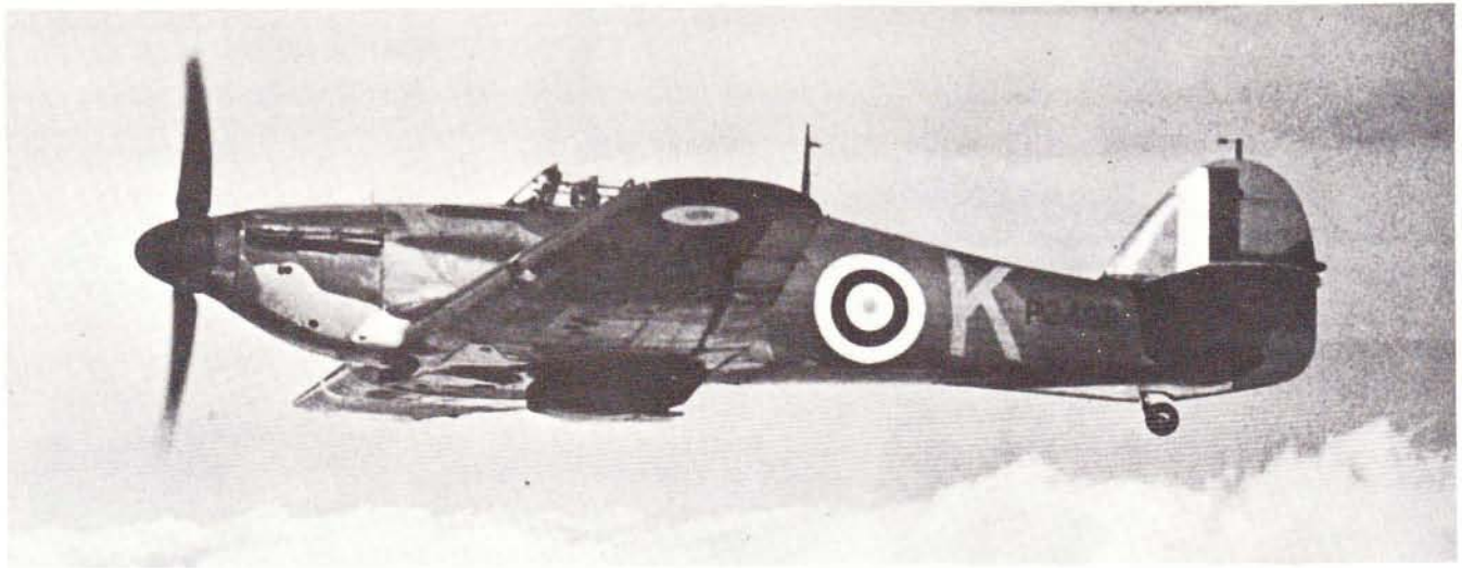
Figs. 14 & 15 Hurricanes of No 85 Squadron above cloud-covered England towards the end of the Battle of Britain. Note how the "Sky" under-surface colour has been extended up the side of the nose of P3408 VY-K.
