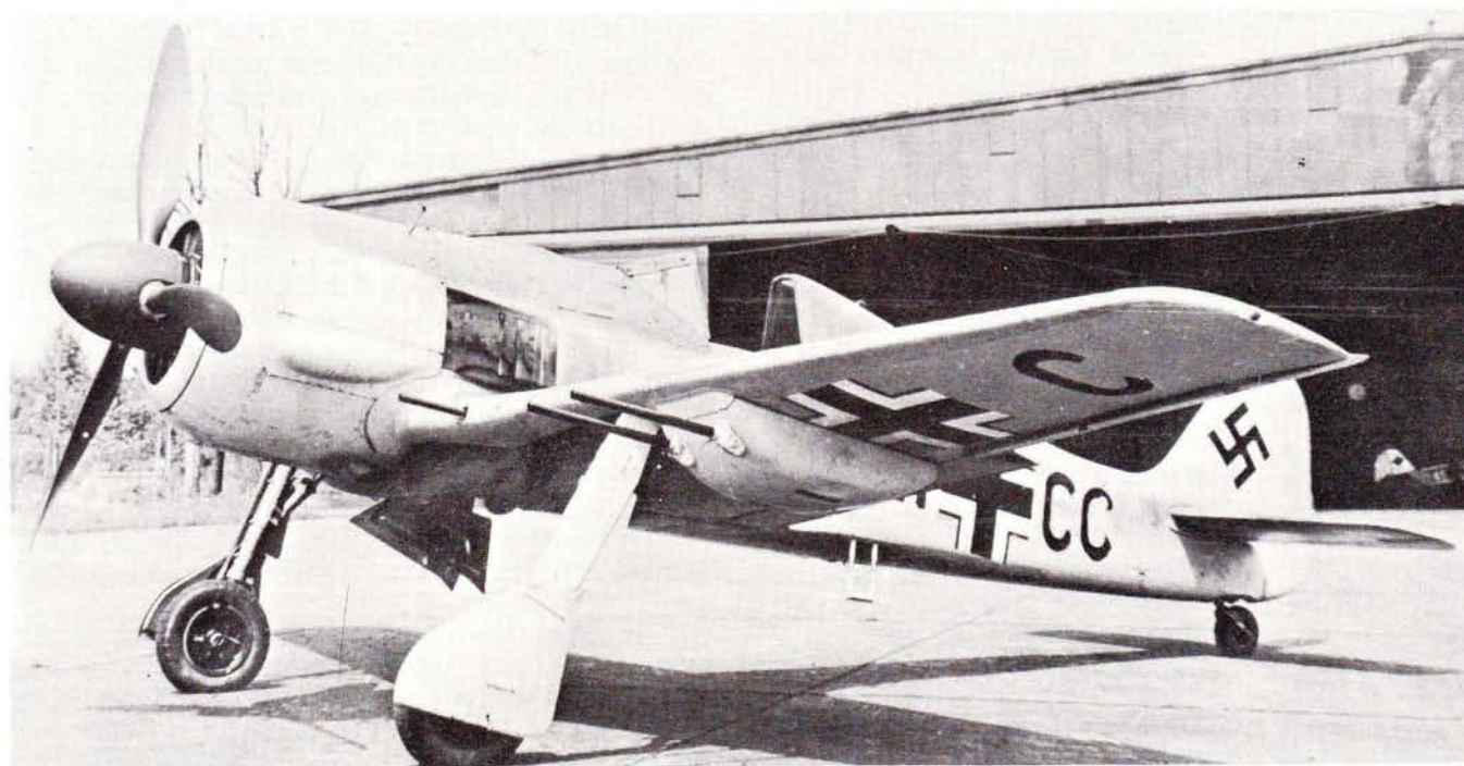
Fig. 29 A-5/U12 W Nr 813, carrying four 20mm MG 151 cannon in twin underwing packs, was used for armament trials.
