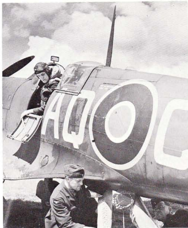
Fig. 21 Ground crews load a dinghy and a food container into the chutes in the belly of Spitfire IIC P8131 AQ-C of No 276 Air-Sea Rescue Squadron early in 1943.
