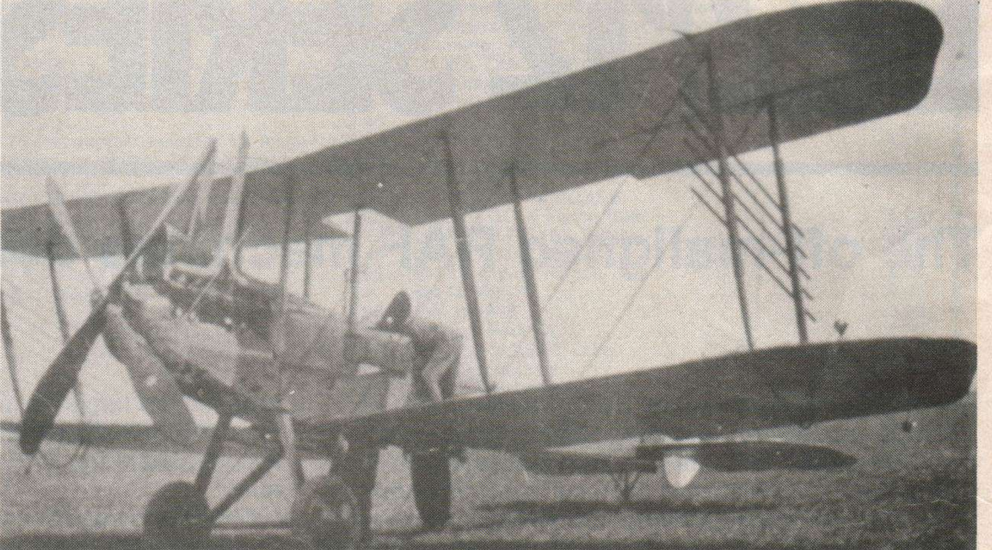
4. BE12 with ten rocket tubes, Holt flare brackets and navigation lights photographed at Spittlegate in 1917.
