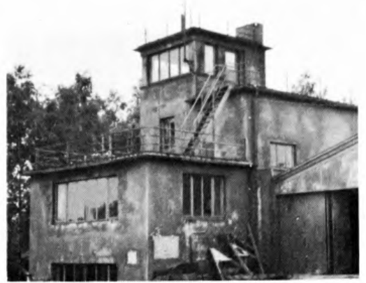
Control Tower at Oerlinghausen.
