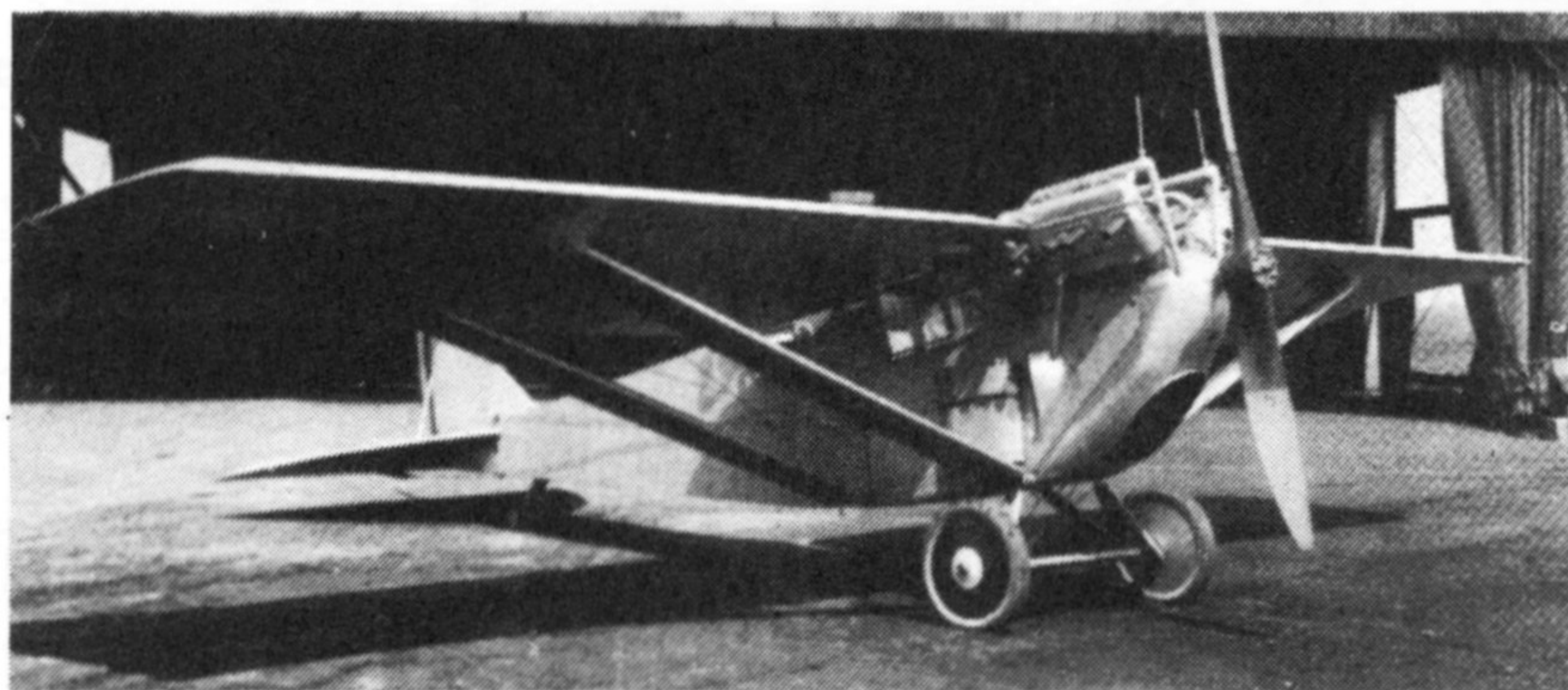
Lifting strut wing braces designed for the M-8 were a breakthrough that has been carried over into lightplane designs of current manufacturing.
