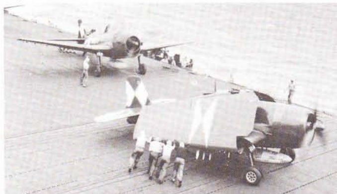
F6F-5s on the deck of the USS Essex in April 1945. Note the belly tanks and underwing rockets on both airplanes, and the deck crew manually folding one plane's wing (center). The various white markings shown here were adopted in late 1943 to identify airplanes from different aircraft carriers.
