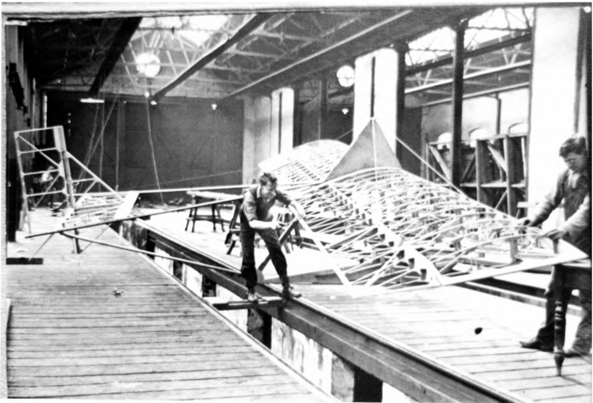
Assembling the Primary in the Scarborough tram sheds. The inadequate working conditions are obvious. ( Slingsby collection )
