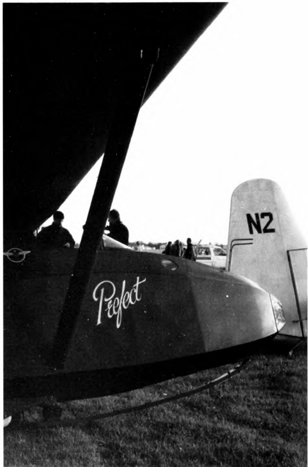
G-ALPC, the second Prefect built, is shown here at Dunstable in 1950. Note that the airbrakes were of the old DFS pattern. On later Prefects these were replaced by the vertical 'parallel-ruler' brakes of Schempp-Hirth type. In the left background is the wing of the two-seat Hawkridge Venture G-ALMF. ( Slingsby collection )
