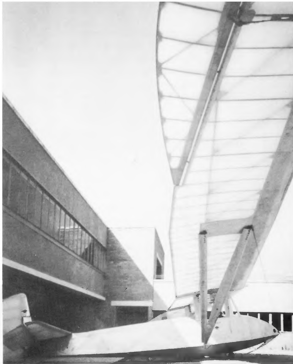
The Falcon 3 at the hangar door at Dunstable. The building was designed by architect and glider pilot Christopher Nicholson and is now the subject of a preservation order.
