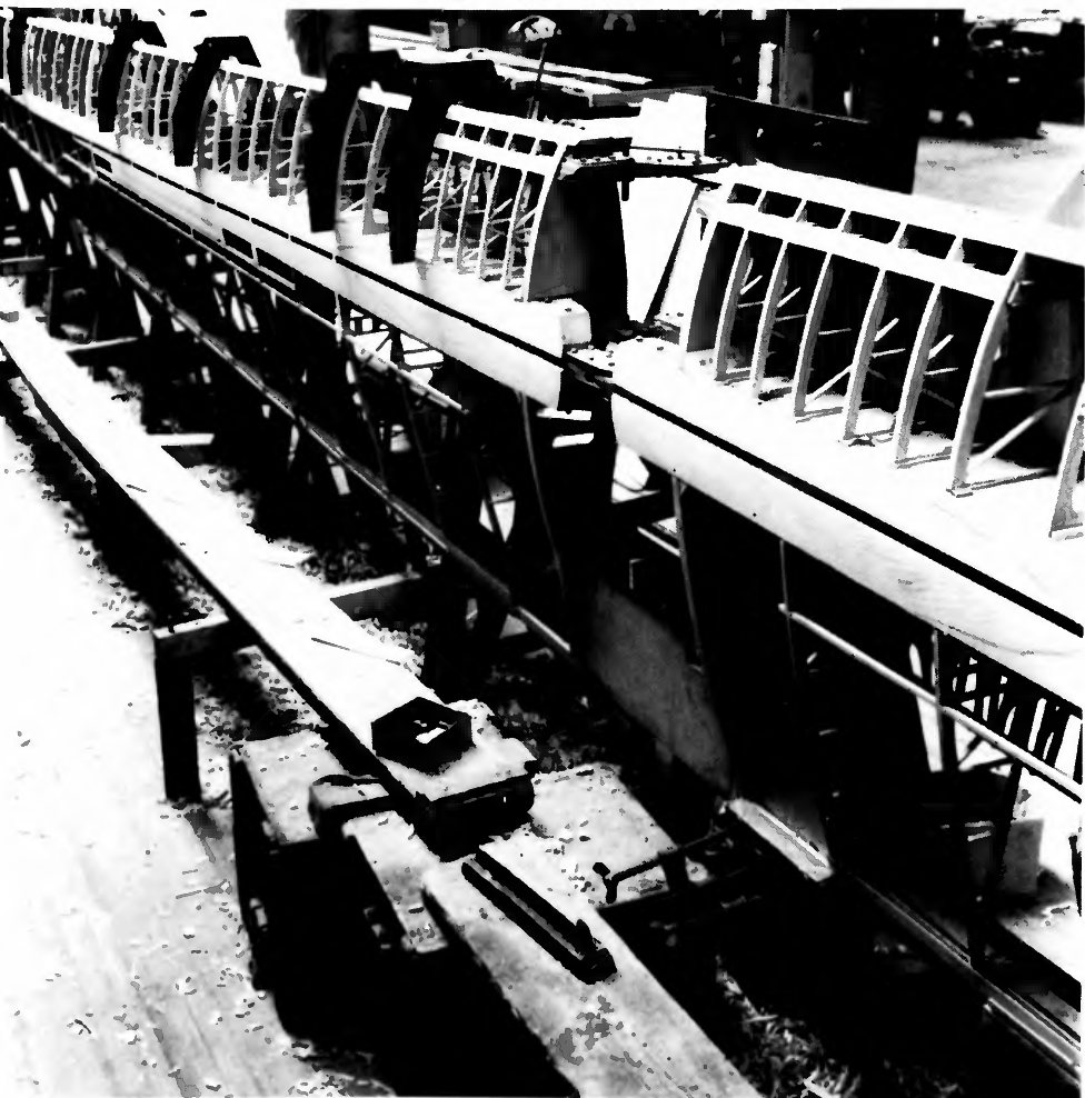
Construction of the Dart 15 at the factory. Note the templates used to check the ribs for accuracy, and the very heavy twin spruce spar on this early production aircraft. ( Slingsby collection )
