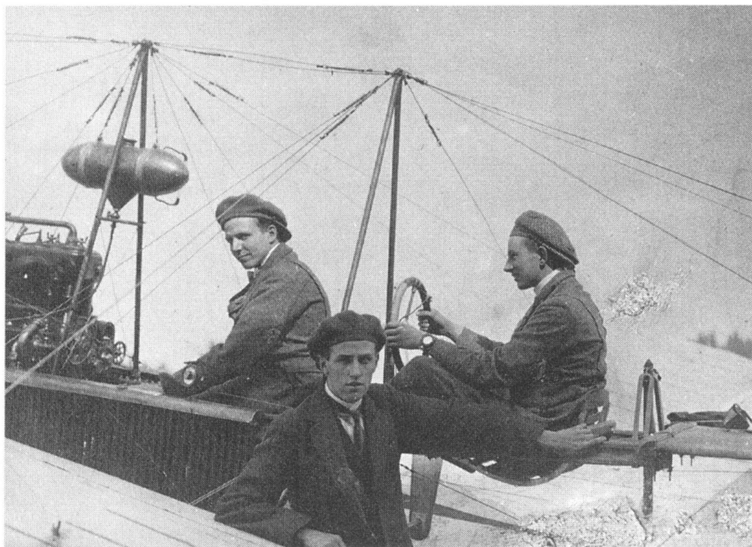
Fokker in the rear 'cockpit' of his third Spinne with Fritz Cremer in the front and Th. Reinhold standing. The engine is the 50hp Argus. Frank Cheeseman
