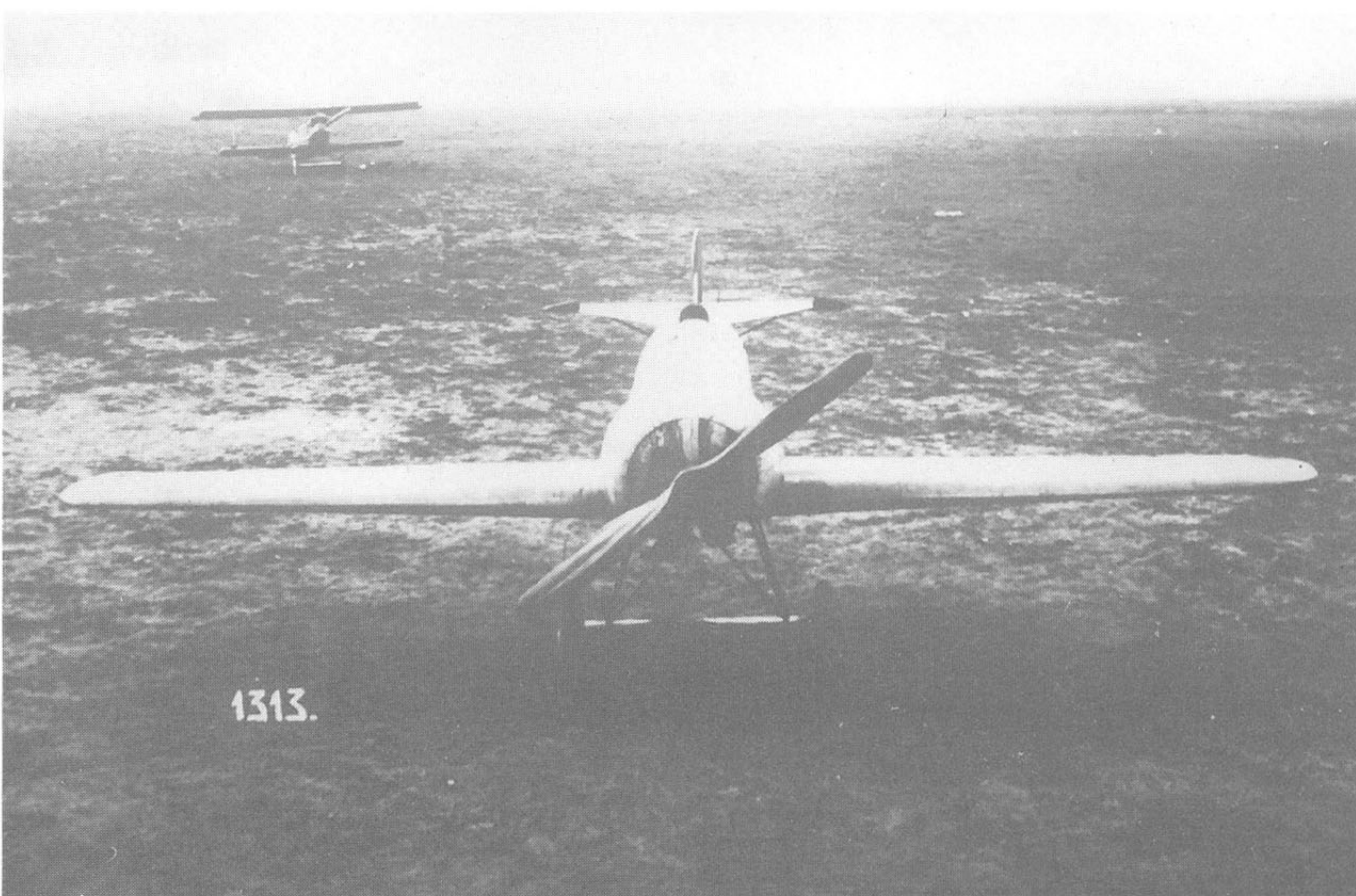
(Above left) Fokker V.25 fitted with a 110hp Oberursal UR.II rotary engine. Cross and Cockade International
