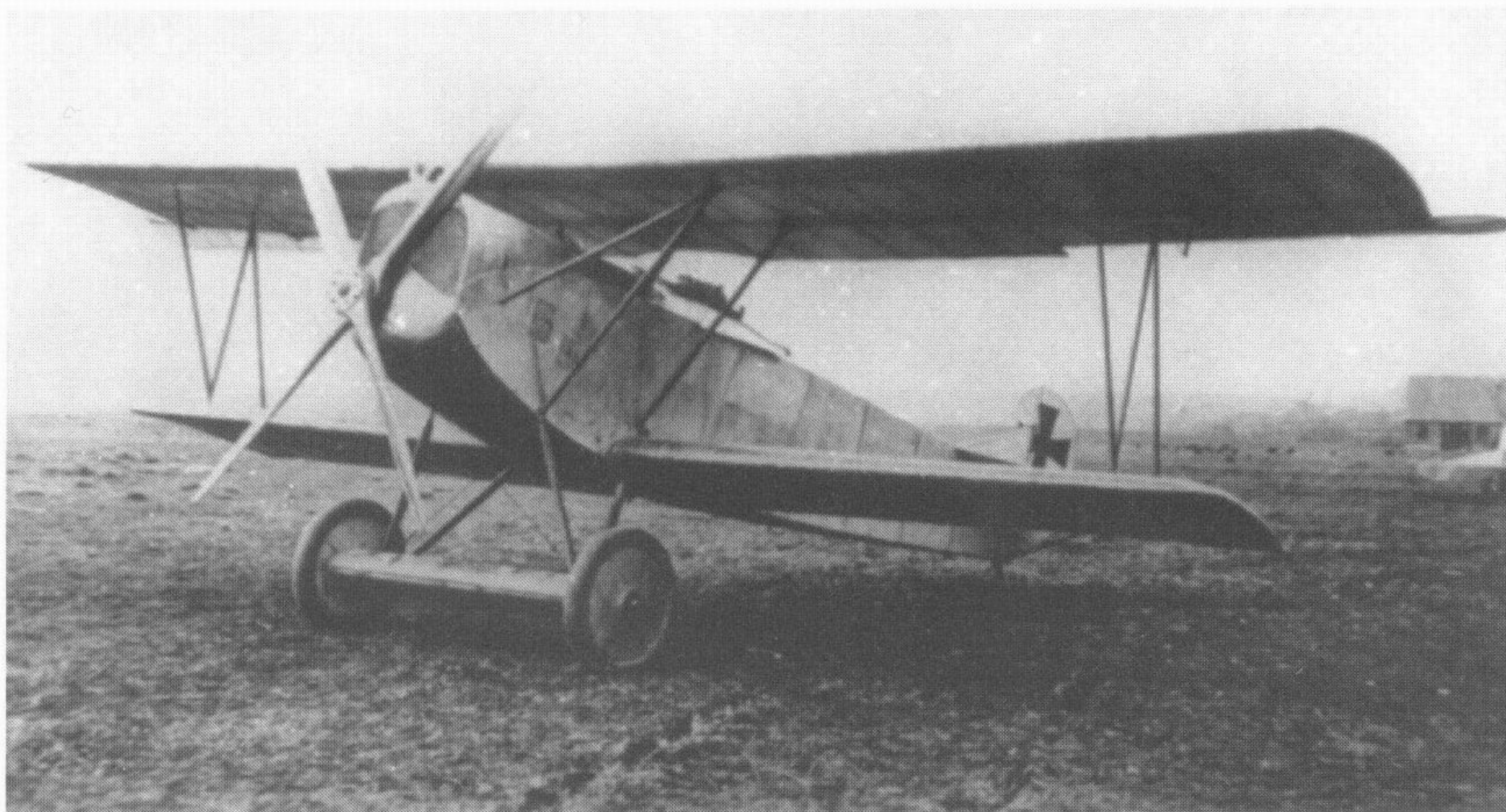
V.22 fitted with a Jaray four-bladed propeller. Cross and Cockade International
