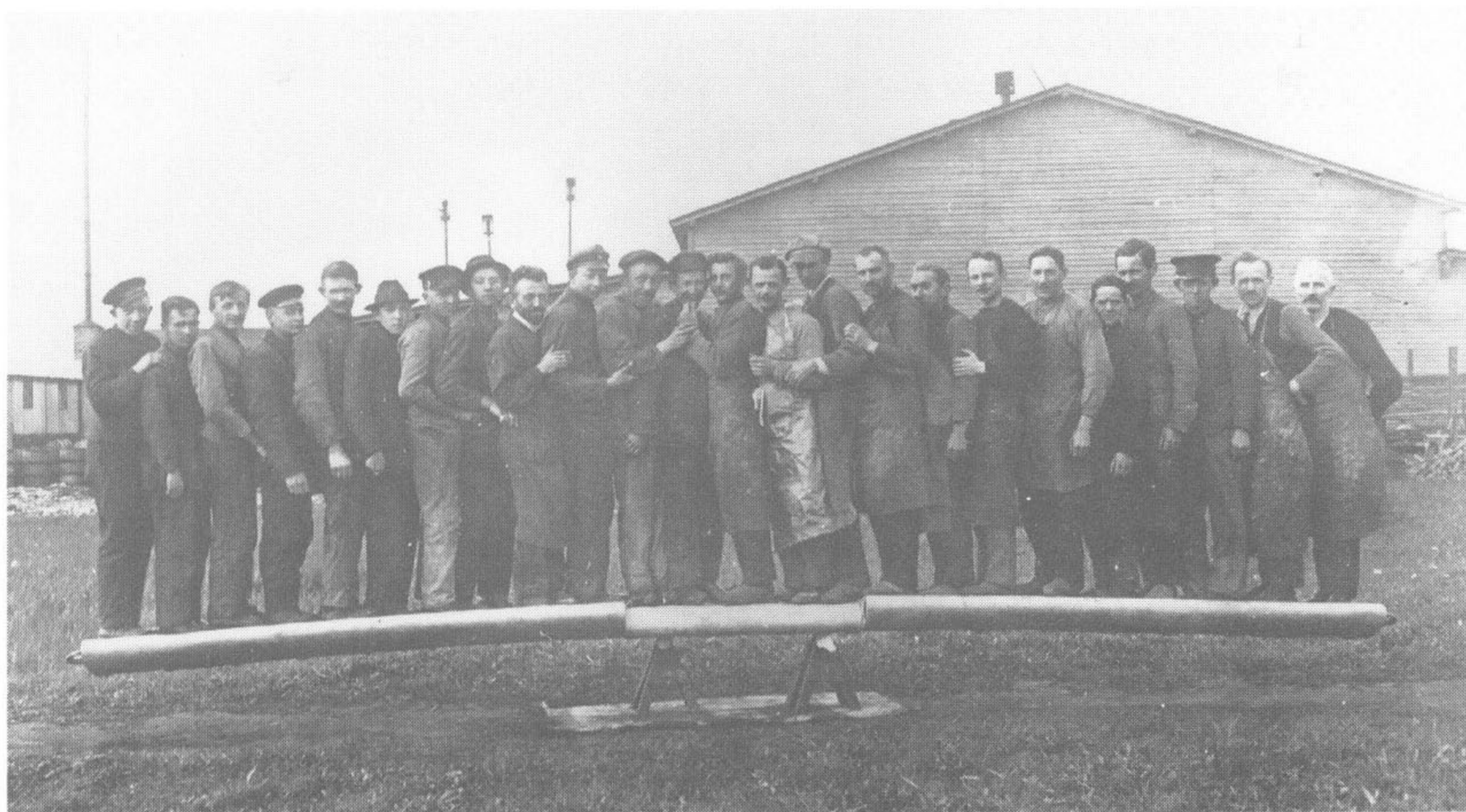
A typical Fokker-style demonstration of strength. The wing is that of either a V.4 or V.5. Peter Grosz
