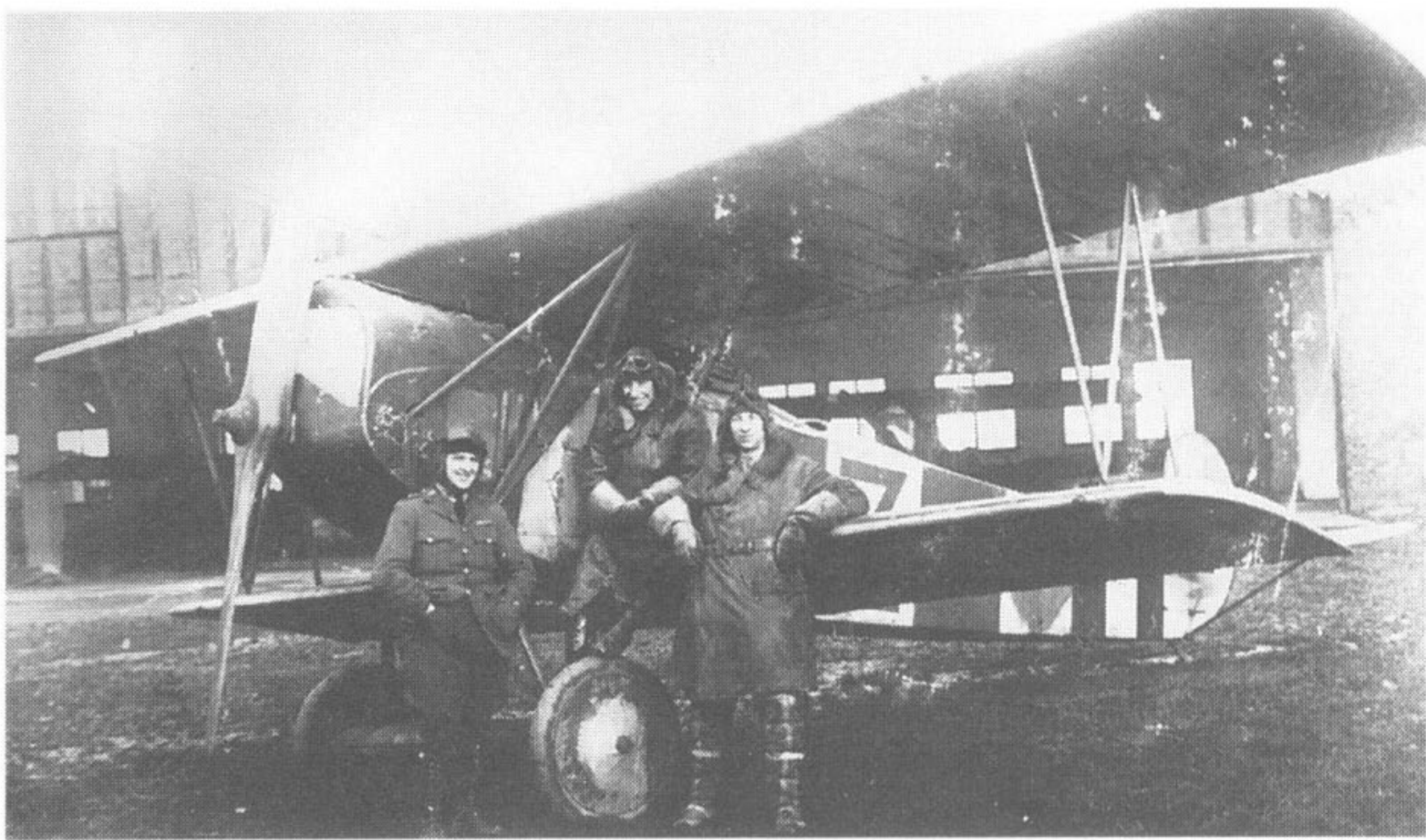
(Above) Fokker D.VII 501/18 seen with RAF personnel at Nivelles after the Armistice. The small quick-release spinner suggests that this was fitted with a BMW engine. Cross and Cockade International
