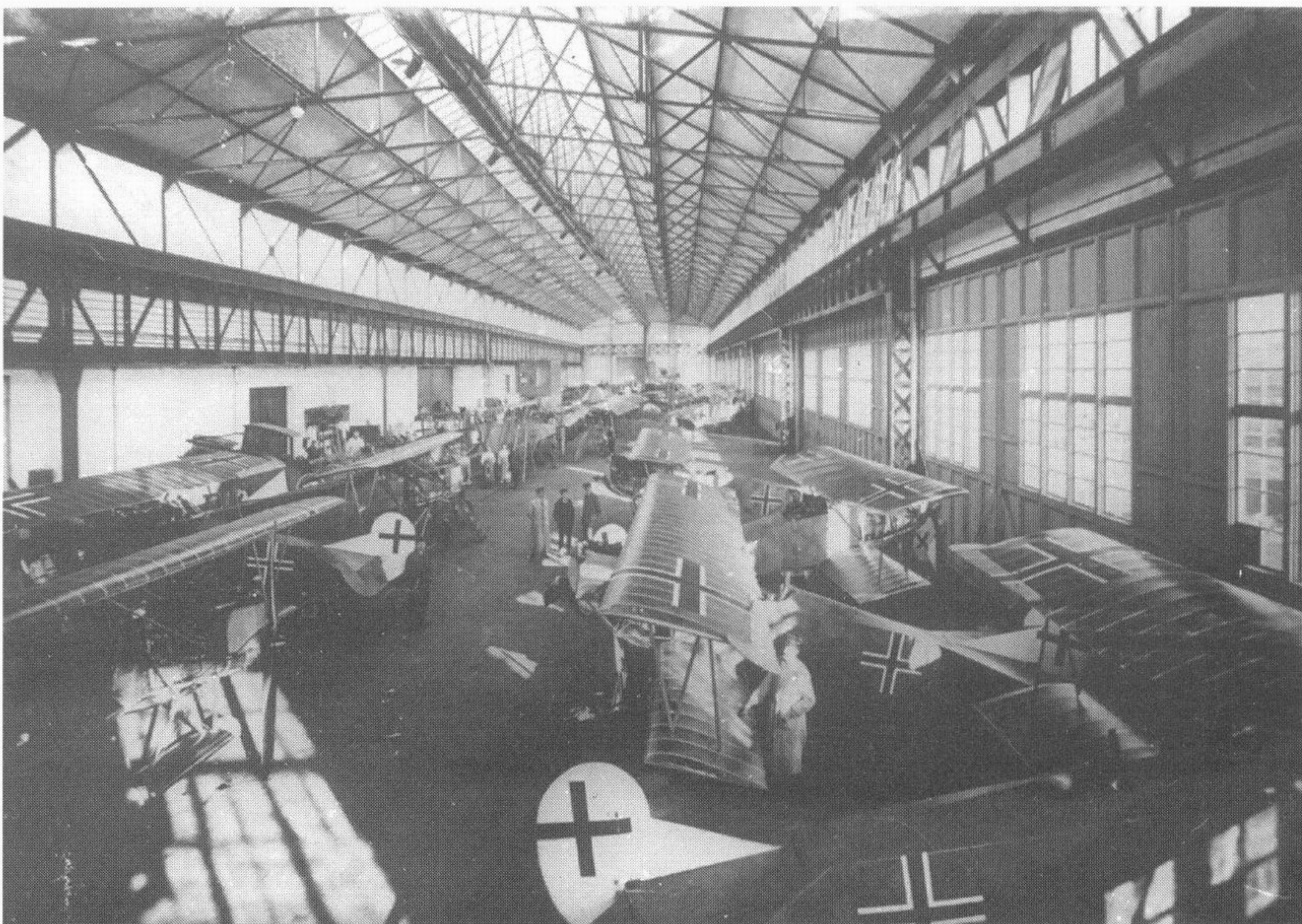
(Right) Assembling a Fokker D.VII at Schwerin. Cross and Cockade International
