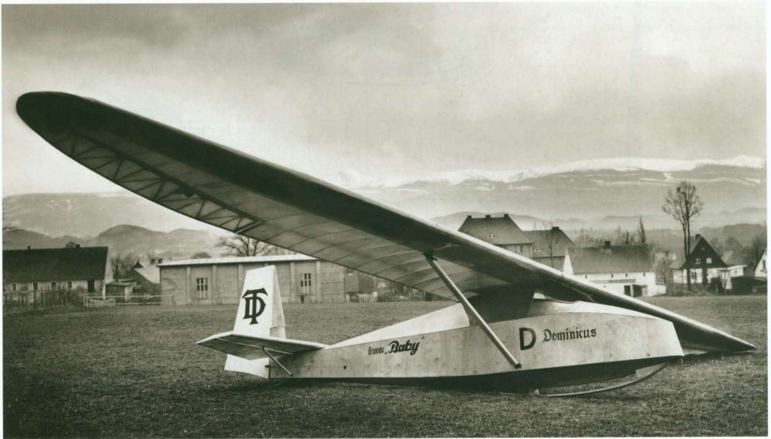
Above: The Grunau Baby 1 had a straight backed fuselage and tall rudder.
