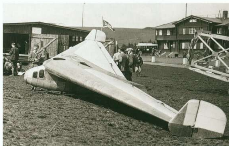
Above and right: Lippisch went on to develop many more tailless aircraft. The Delta I was test flown as a glider by Günther Groenhoff at the 1930 Rhön, though not competing. It was subsequently converted to power and flew in 1931. It was difficult to handle on take off and crashed severely in 1933.
