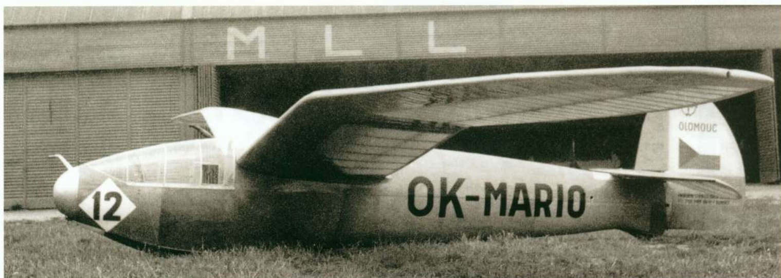
Above and right: The Duha 2, OK - Mario, designed and flown at the Internationals by J Chlup, was a much changed version of the Duha 1. It was a fifteen metre sailplane with a wing of pronounced 'gull' form, and a contoured transparent canopy. Chlup did not make a score. It has not been possible to make an accurate drawing of this type.
