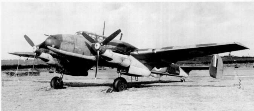
Three views of Messerschmitt Bf 110 C-5 5F+CM, W.Nr. 2177, of the 4.(F)/14 taken after being forced down over southern England on 21 July 1940 by Hurricanes of 238 Squadron. Finished in an upper camouflage scheme of 02/71 with 65 under surfaces, a mottle of 02/71 or 70 was applied in varying densities and height along the blue of the fuselage sides and to both sides of the fin/rudder assemblies.
