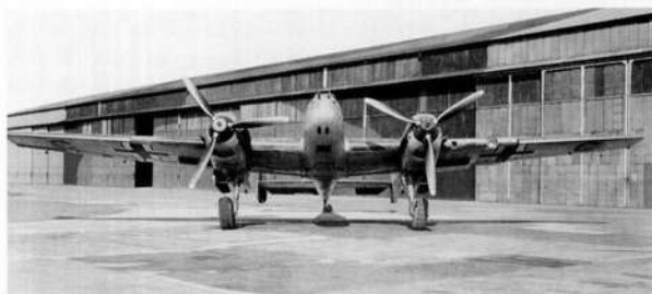
Three views of Messerschmitt Bf 110 C-5 5F+CM, W.Nr. 2177, of the 4.(F)/14 taken after being forced down over southern England on 21 July 1940 by Hurricanes of 238 Squadron. Finished in an upper camouflage scheme of 02/71 with 65 under surfaces, a mottle of 02/71 or 70 was applied in varying densities and height along the blue of the fuselage sides and to both sides of the fin/rudder assemblies.
