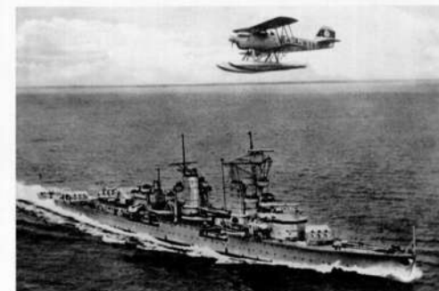
A pre-war view of Heinkel He 60c, 60+B11 of the 1./KüFlGr. 106 flying over the cruiser 'Köln' during exercises in the Baltic Sea. Clearly visible between the funnels of 'Köln' is the amidships mounted aircraft catapult in the stored position.
