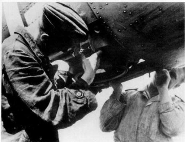
Technicians carrying out the installation or removal of a camera from the fuselage bay of an unidentified aircraft believed to be either a Do 17 or Ju 88.
