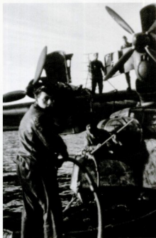
These three photographs are from a series that was taken of a Blohm and Voss Bv 138 C-1 rendezvousing with and refuelling from an unidentified U-boat in far northern waters. It is thought however, that as the aircraft is fitted with FuG 200 Hohentwiel search radar, the photographs were probably taken in early 1944.
