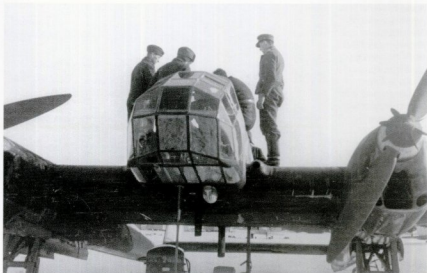
Left: Luftwaffe personnel at an unidentified airfield on the Eastern Front inspect a badly damaged Focke-Wulf Fw 189 A-1, 4E + TK of the 12.(H)/13 in late 1943. Although fitted with the standard upper dorsal armament of the A-1, the tail position is fitted with the later MG 81Z installation of the A-2, and the unit code letters of 4E, although barely visible, have been applied in accordance with the change ordered in mid-1943.
