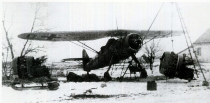
A Henschel Hs 126, 4E-DM of the 4.(H)/13 sits awaiting an engine change at an airstrip in the area of Federowka during the mid-winter of 1941-42. It is of interest to note that while one BMW engine is slung beneath a tripod hoist, a second sits on a small sled – a most practical method of transporting engines over a short distance in the prevailing weather conditions.
