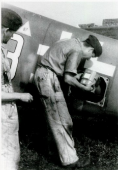
Staffel Bildstelle personnel of the 1./NAGr. 2 are seen here fitting one of the paired Rb 12.5/7x9 cameras into the rear fuselage of a Bf 109 G-8 of the Staffel. Formed in Russia from the 4.(H)/10 on 1 March 1943, the Staffel disbanded at Olmütz (now known as Olomouc, in the Czech Republic) in March 1945.
