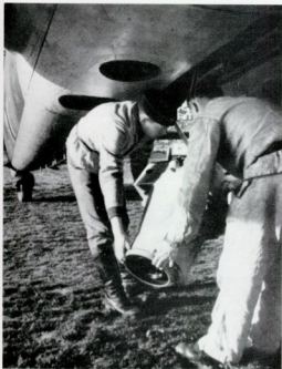
Possibly taken at Witebsk, Russia, in the late summer of 1941, these two undated views show Bildstelle personnel of the 2./F1/122 preparing to install three Rb type cameras into Junkers Ju 88 D-2, F6-1K.
