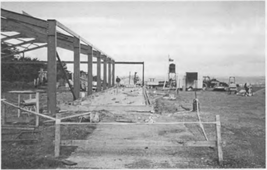
The new buildings going up
