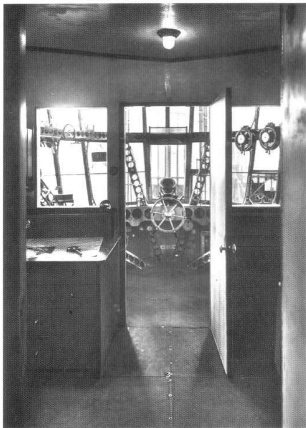
36 Below: A view into the control car of the LZ127, Graf Zeppelin. The marine ancestry of the vessel is apparent in the steering wheel, chart table and windows akin to a ship's bridge
