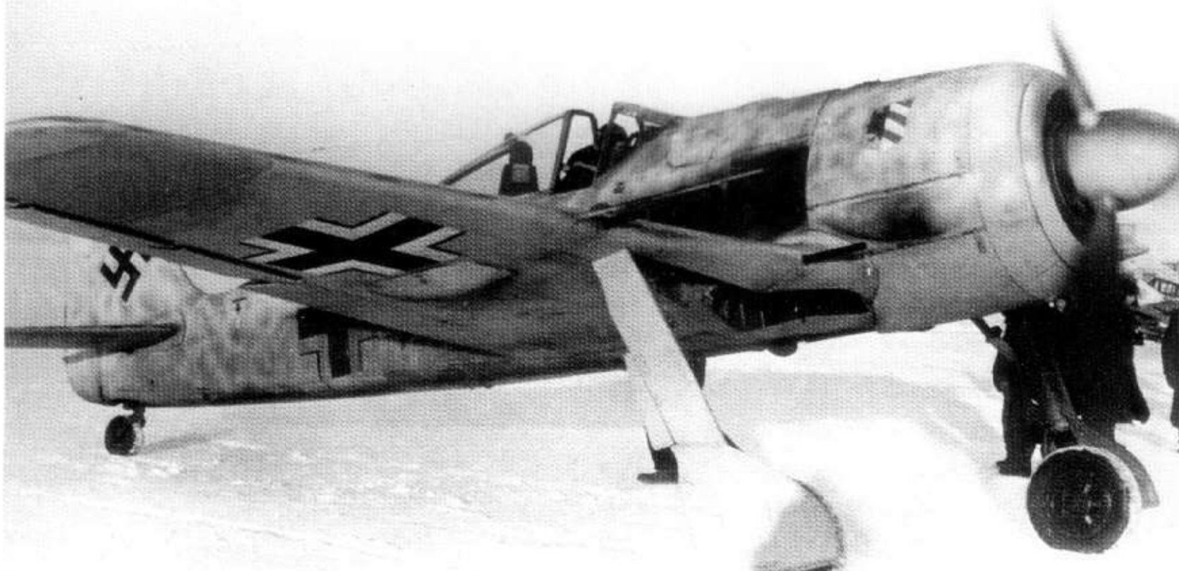
201 Above: An Fw 190A-4 of I./JG 54 starts up at Siverskajya in winter 1943. The spray painter has given a slightly mottled effect to the temporary white finish which enhances the camouflage effect. It can be seen that the wheel bay, wheel cover interior and landing gear were painted in 02
