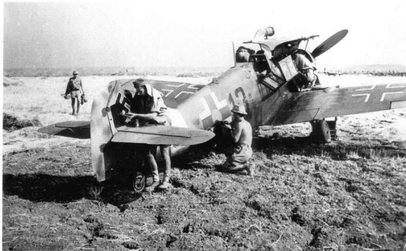
150: A Messerschmitt Bf 109, 'Black 13', having its national markings changed by South African personnel. This may be the Bf 109F trop which was captured by No. 4 Squadron SAAF at LG12 in late December 1942. It appears to wear the unusual 'saw-tooth' edged 74/75 camouflage pattern applied to a number of the reconnaissance variants of the Bf 109
