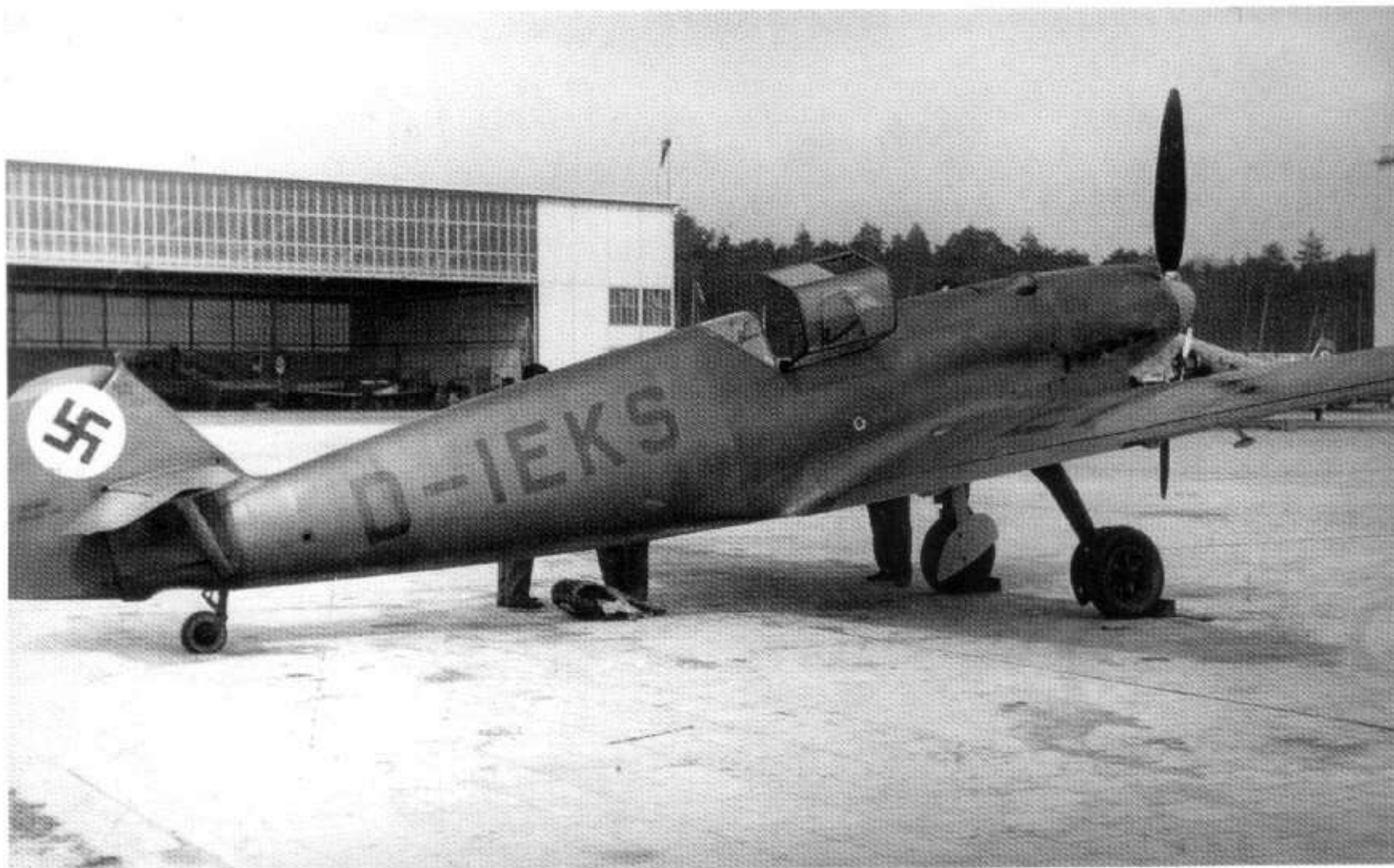
48: This is the Messerschmitt Bf 109V-5 (B-02) in 1936, fitted with a variable-pitch VDM propeller. It was later sent for trials with the Legion Condor in Spain. Here it wears a Class B1 civilian registration, D-IEKS, on what appears to be low contrast camouflage of RLM 70/71, a portion of the pattern of which can be just made out on the nose below and diagonally forward of the air intake. The spinner appears to be light grey or yellow. While the serial number for this aircraft is recorded elsewhere as 879, the legend 'WNR 320' can be made out on top of the fin in the original photo
