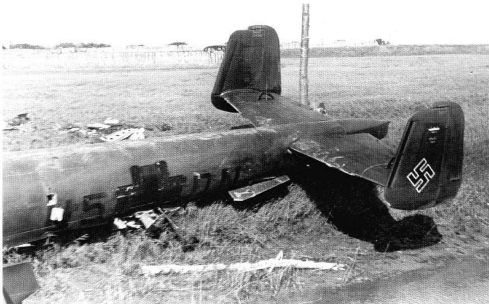
221: Another view of Lt Dolenga's Dornier Do 217E-1, WNr 0069, U5+DN, of 5./KG 2, (see photo 103) in the low contrast 72/73 camouflage. The aircraft had received a removable night camouflage on the undersurfaces which also obscured the fuselage markings. The Balkenkreuz was not repainted with the special marking colour 77 and the swastika had remained untouched. The fin sports two ship kill markings
