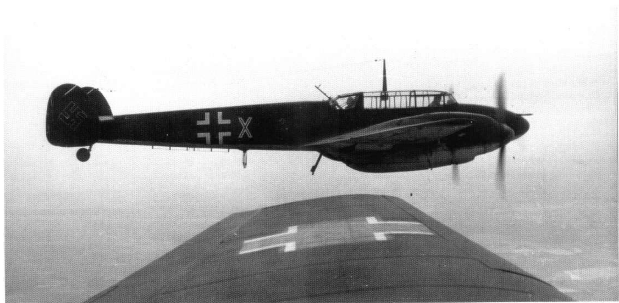
232 Below: A Bf 110C-2 of Stab I/LG 1, L1+XB, (green 'X'), finished in standard 70/71/65. Many early Luftwaffe night fighters bore this scheme. Note the glossier finish to the wing cross in the foreground
