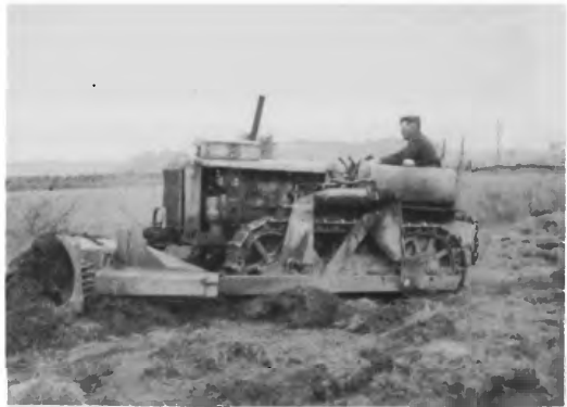
Levelling the airfield for aero-towing
