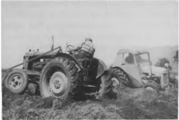
Levelling the site for the hangar.
