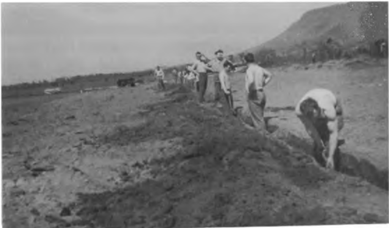
Digging the foundations for the hangar
