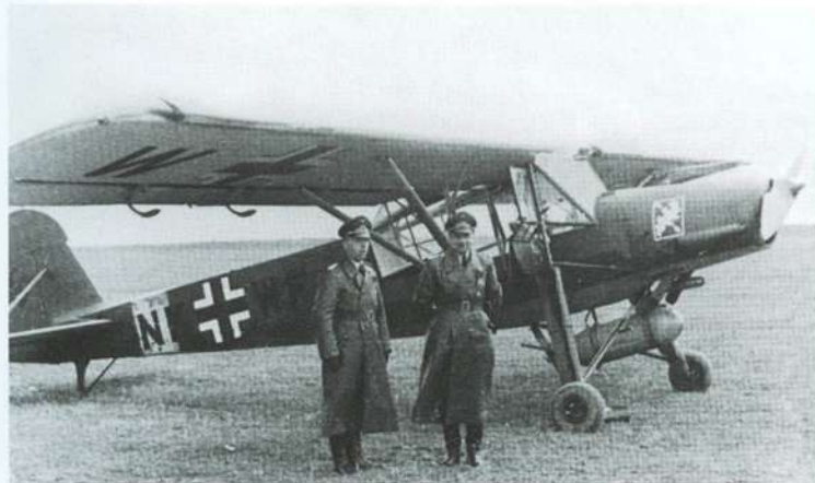
This Fieseler Fi 156 C 'Storch' belonged to the Flugber./Luftgau-Kdo.Moskau and was photographed in Russia during 1942. Only the letter 'D' of the Stammkennzeichen can be seen in the photograph (?D+??). It had a standard factory 70-71 splinter upper surface camouflage scheme with the rarely seen emblem for this unit.
