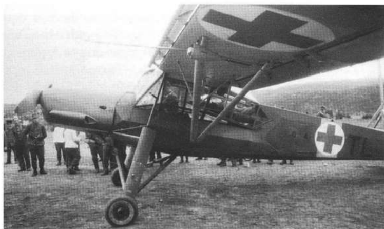
This 'Storch' had tandem landing gear. It was Fi 156 D-1/trop, W.Nr. 5700, GB+XT, which was assigned to Sanitäts Flugber.8 in Finland during the summer of 1944. The aircraft had a standard factory 70-71 splinter scheme with a yellow fuselage band and underwing tips.
