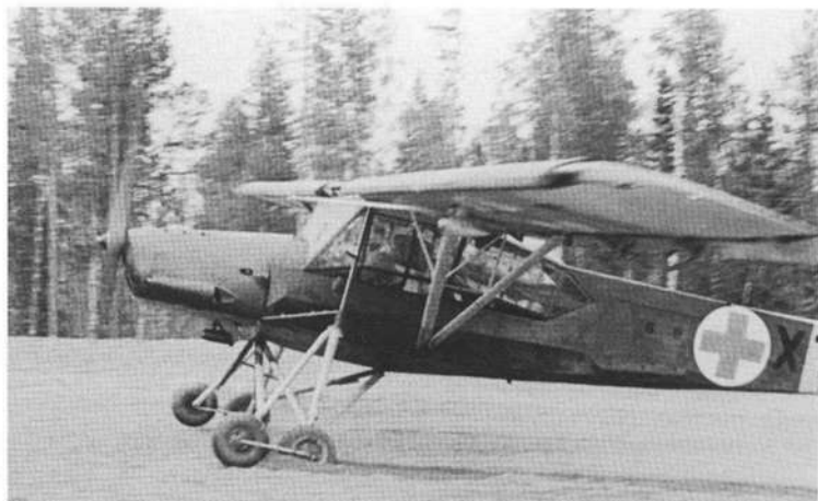
This 'Storch' had tandem landing gear. It was Fi 156 D-1/trop, W.Nr. 5700, GB+XT, which was assigned to Sanitäts Flugber.8 in Finland during the summer of 1944. The aircraft had a standard factory 70-71 splinter scheme with a yellow fuselage band and underwing tips.
