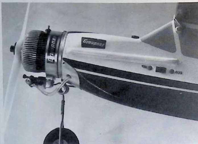
The Schaegg-designed experimental Wankel engine of 1967 installed in the Graupner "Taxi" model in which it was publicly demonstrated in Europe at that time. (Photo: Courtesy Johannes Graupner)
