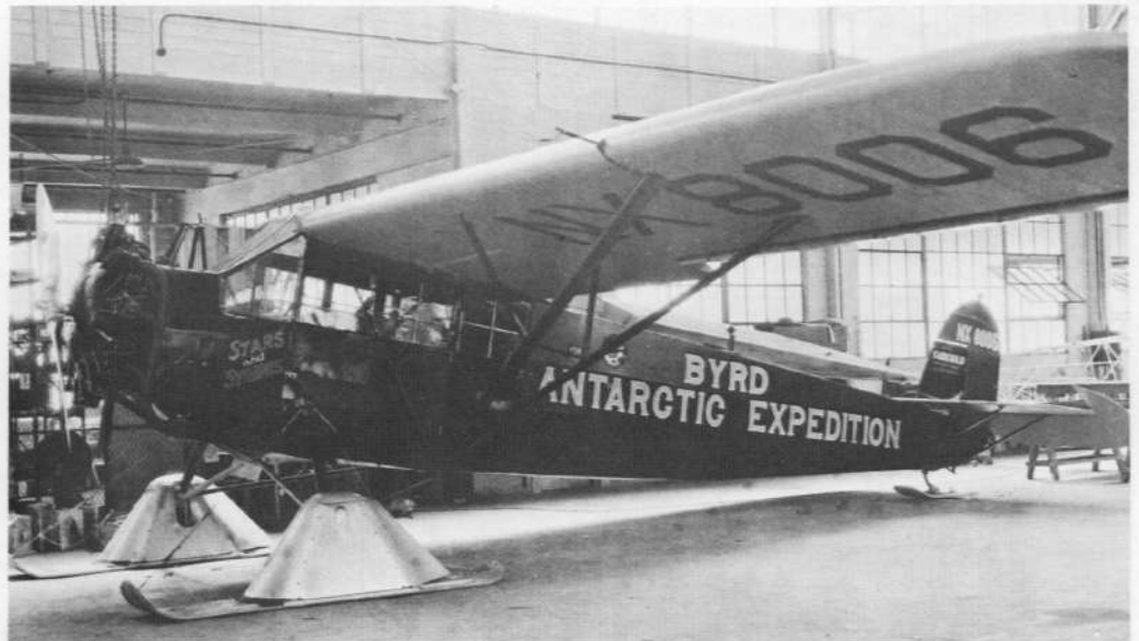
"Stars and Stripes" during final assembly at the Fairchild factory. Note wing support strut for wing in folded position.
