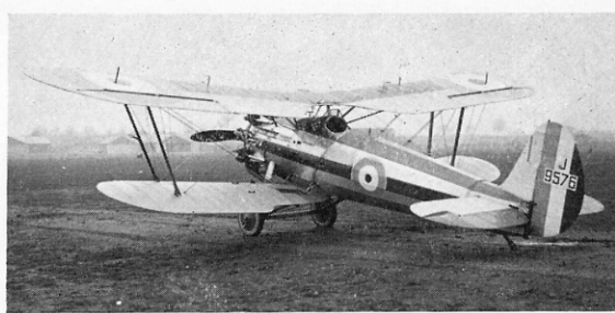
Left: Prototype Bulldog II, c/n 7235, serial J9480. First flew on 21st January 1928. Right: 11th production Bulldog II, c/n 7332, serial J9576, in No. 3 Squadron colours. No. 3 was the first squadron to operate Bulldogs. Note amended fin shape.
