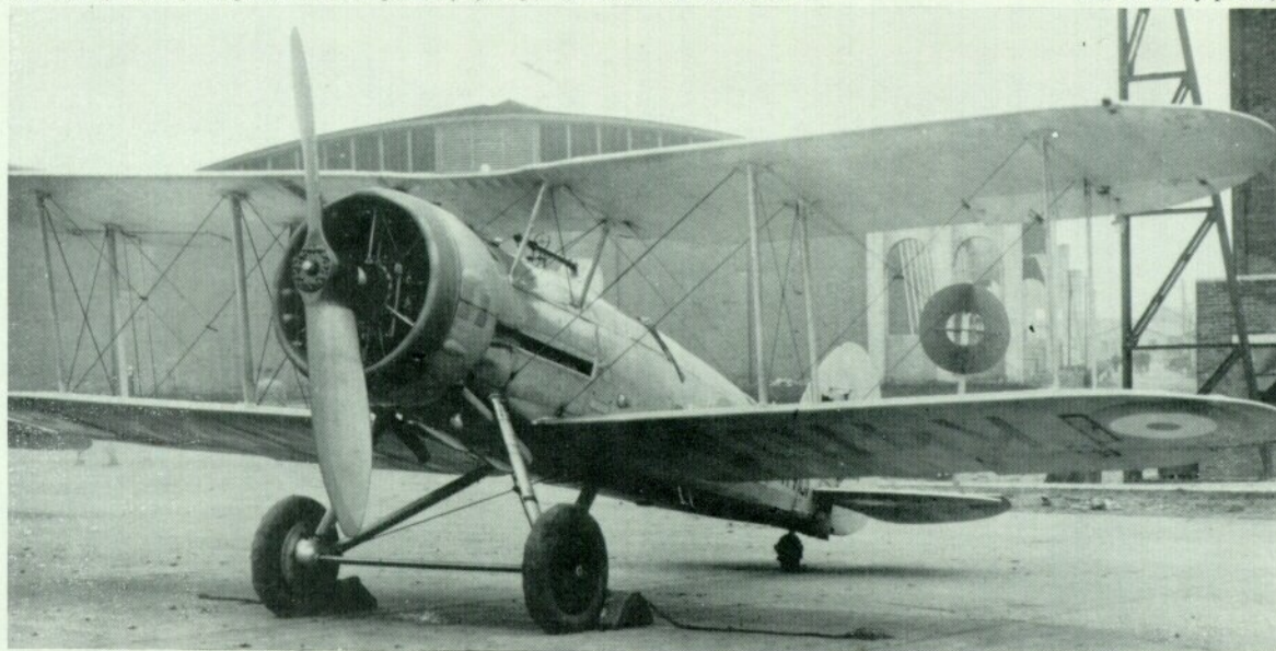
Gauntlet I, K4101, was fitted with low pressure tyres for service in the Middle East.
