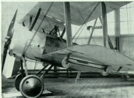
Probably used in experiments in taking off from ships, this Beardmore-built Pup had two grooved wheels under each lower wing.
