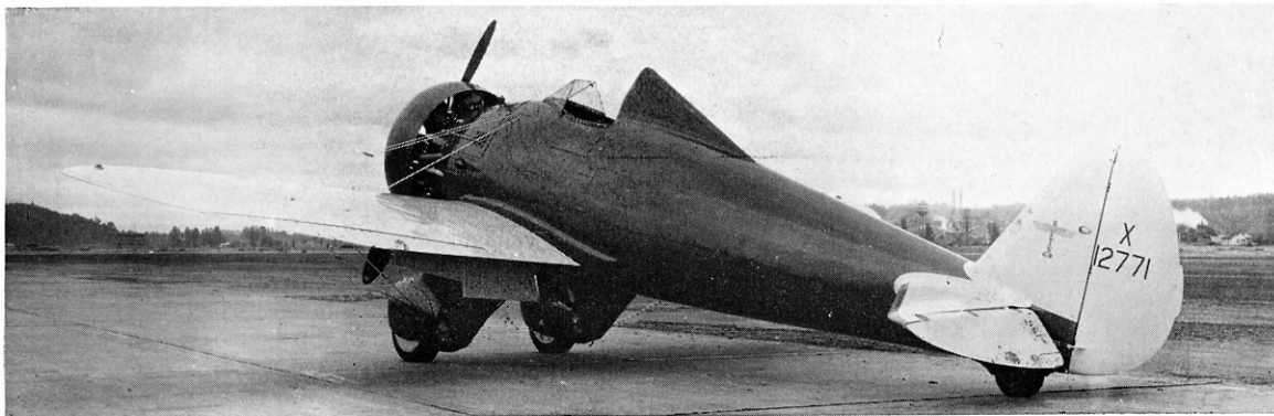
First Boeing Model 281, export version of the P-26A. This aircraft was used by Boeing to develop a flap design that was eventually fitted to all 26As and Cs. (Photo: Boeing)
