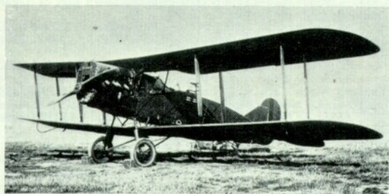
Above: Possibly a SABCA-built Bristol F.2B, this was No. 45 of l'Aéronautique Militaire Belge, with 300-h.p. Hispano-Suiza engine, oleo undercarriage and horn-balanced rudder. Below: One of twelve new-built Bristols supplied to Spain in 1924 with 300-h.p. Hispano-Suiza, oleo undercarriage and Frise ailerons.
