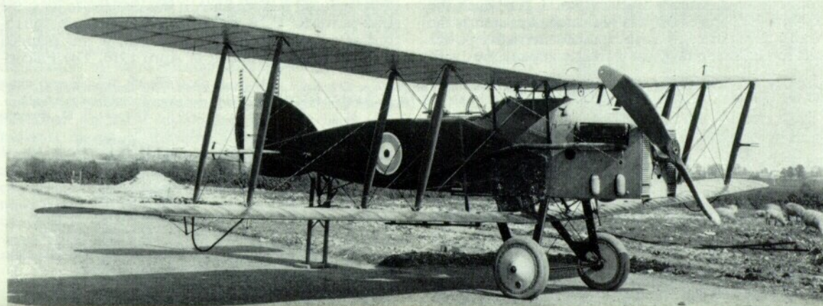
Above: The final Arab installation, using a radiator of the shape designed for the 300-h.p. Hispano-Suiza, here seen on F4640. (Photo: Imp. War Mus.)
