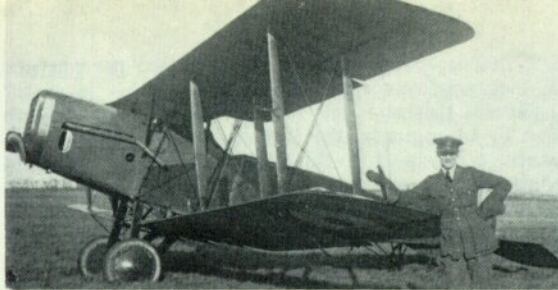
Left: A few Falcon-powered Bristol F.2Bs had radiators of increased area that substantially altered the shape of the nose. This one was photographed at the Isle of Grain shortly after the Armistice; another was at Cranwell in August 1919. Right: In the early post-war years experiments were conducted with free-flying target gliders, one of which is seen here on a Bristol F.2B. A larger type of glider was launched from a Westland Walrus.
