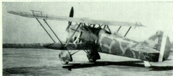
The final production variant in the series was the C.R.32quater, which remained in production until the autumn of 1939. (Photo: G. Apostolo)
