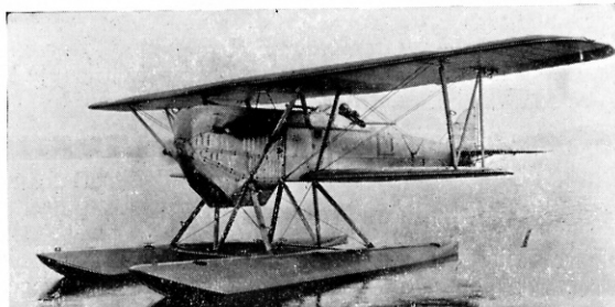
Left: Major production model of FB series was FB-5, Boeing Model 67, which could be operated as a landplane or a twin-float seaplane. Right: F2B-1, Boeing Model 69, was improved PW-9|FB-5 designed for P&W Wasp radial engine. (Photos: U.S. Navy)
