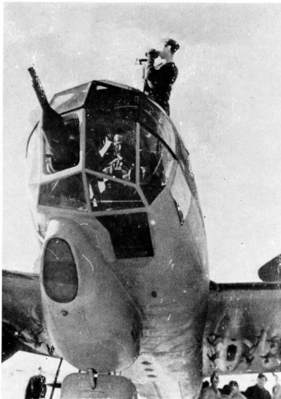
Non-standard Ju 88A-4, with 20 mm. cannon mounted in the nose "glass-house".
