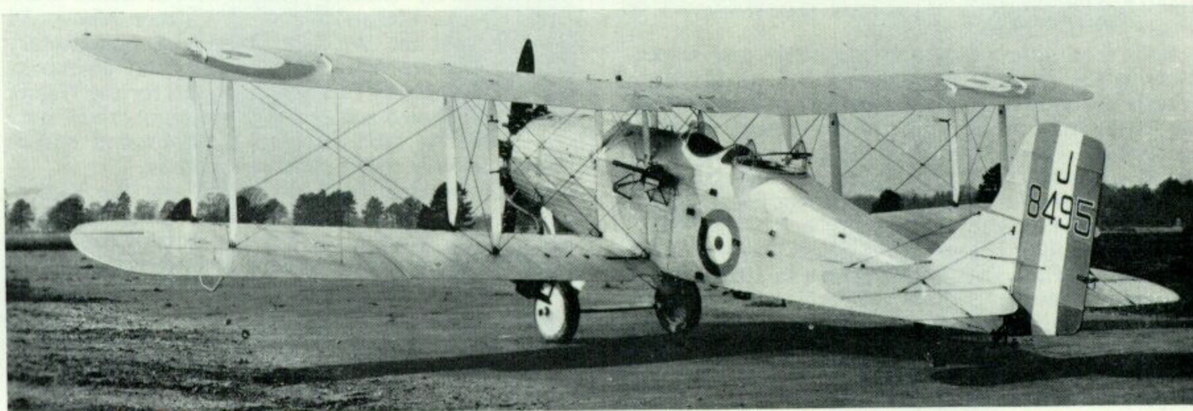
Above: Prototype Wapiti, J8495, with modified fin and rudder, photographed during general purpose aircraft competition at Martlesham Heath (Photo: Air Ministry). Below: J8495 with large fin and rudder and fin fillet, as prepared at Yeovil for the R.A.F. Display, Hendon 1927.
