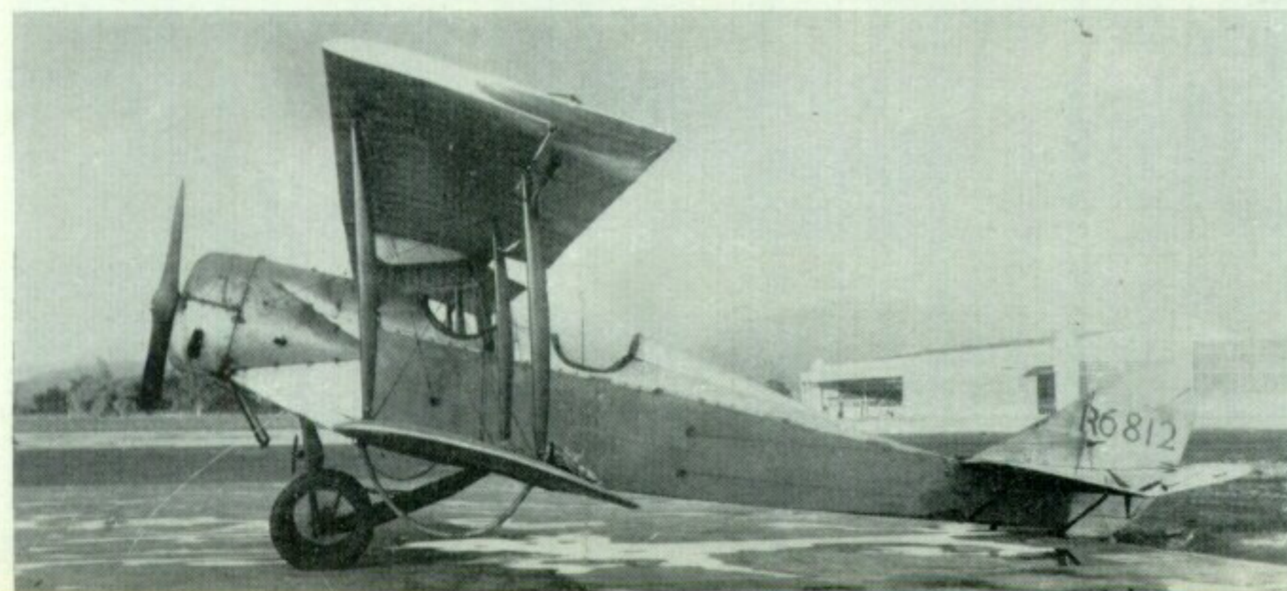
A private owner attempted to improve the performance of this JN-4D by installing a 160-h.p. Gnome rotary engine, clipping the upper wingtip, and adding aileron area to the ailerons.
