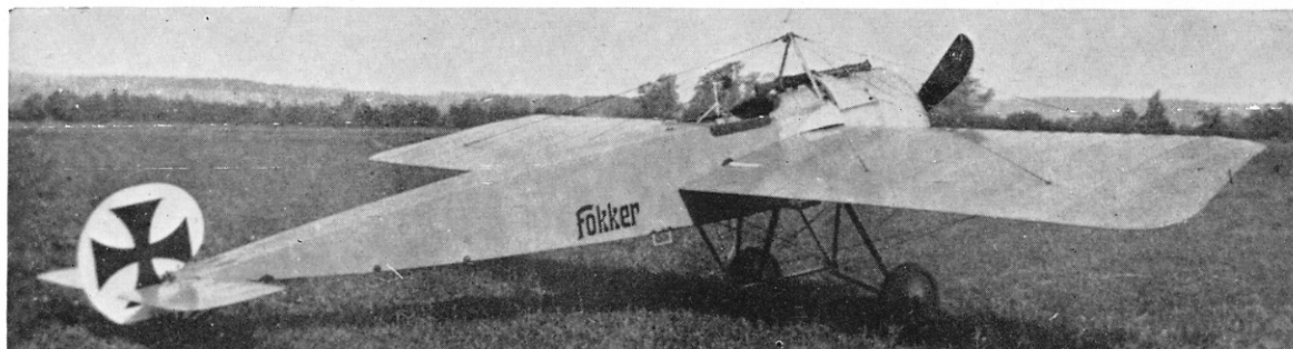
The M.5K/MG with Parabellum gun and head-rest fitted behind the cockpit.
