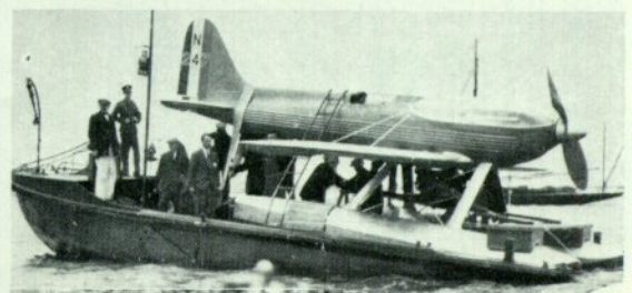
Right: Lighter-borne S.6 being taken out for trials in the Solent in 1929. The aircraft was slid into the water when reaching the starting line.
