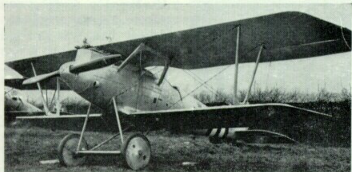
Left: Pfalz D III 4185/17 Justa 5, with red and white fuselage bands photographed at Boistrancourt. (Photo: von Hippel). Right: Early production Pfalz D III in standard ex-works aluminium finish, showing clearly style and location of patee crosses and fuselage serial number. Also to be noted—the black datum on fuselage centre-line extending back from nose. (Photo: Egon Krueger)
