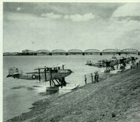
Above: IIF Mk. IVM floatplanes on the Nile. The second aircraft carries the flight colour on its fin. Note also the variations on float structure. Below: IIF Mk. IVs at Khartoum. (In the picture the farthest aircraft is a Fairey Seal floatplane carrying flight leader's fin colours.) (Photos: Ministry of Defence)
