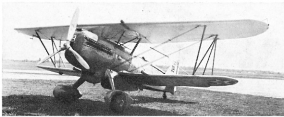
XP-6F showing turbo-supercharger. (Photo: Gordon S. Williams)
