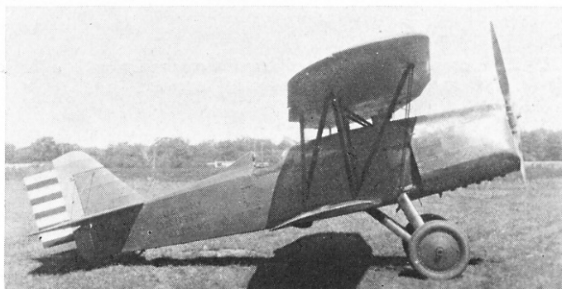
The first P-1 became XP-17 when fitted with Curtiss V-1460 engine. (Photo: U.S.A.F.)
