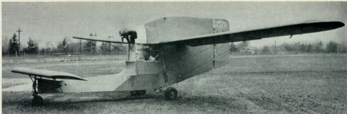
The unique "Ascender" of 1931, a canard design using the wing and powerplant of an Aeronca C-2 ultra-light sportplane. (Photo: Courtesy Joseph P. Juptner)
