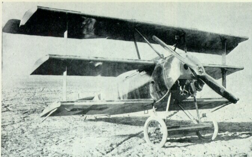
Subject of the official performance trials, Fok. Dr.I 141/17 with the early production ailerons.
