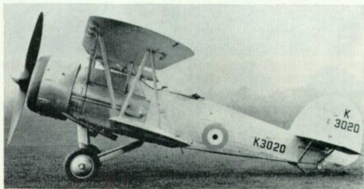
Above and below: The Bristol test-bed Hart, K3020, was flown in turn with short- and long-chord cowlings round Pegasus engines, and with Mercury driving Hamilton 3-blade metal propeller.
