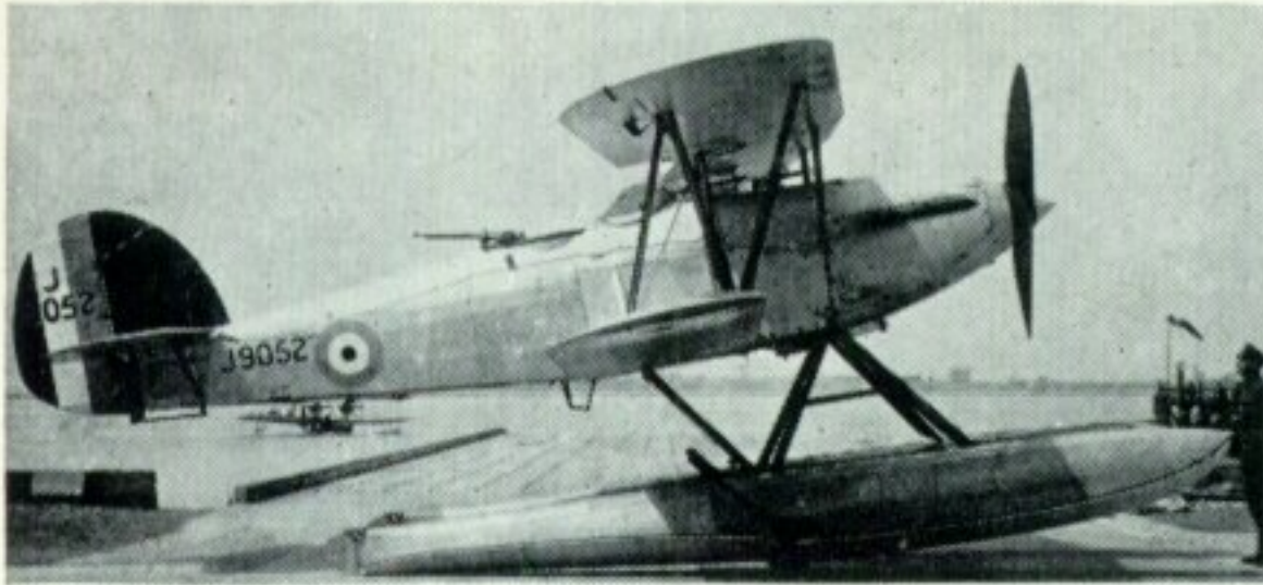
Left: Seen at Felixstowe Marine Aircraft Experimental Establishment, the Hart prototype is here equipped with Osprey floats and tail unit. (Photo: Ministry of Defence, Air Ministry No. 6888B, 6/12/30.)
