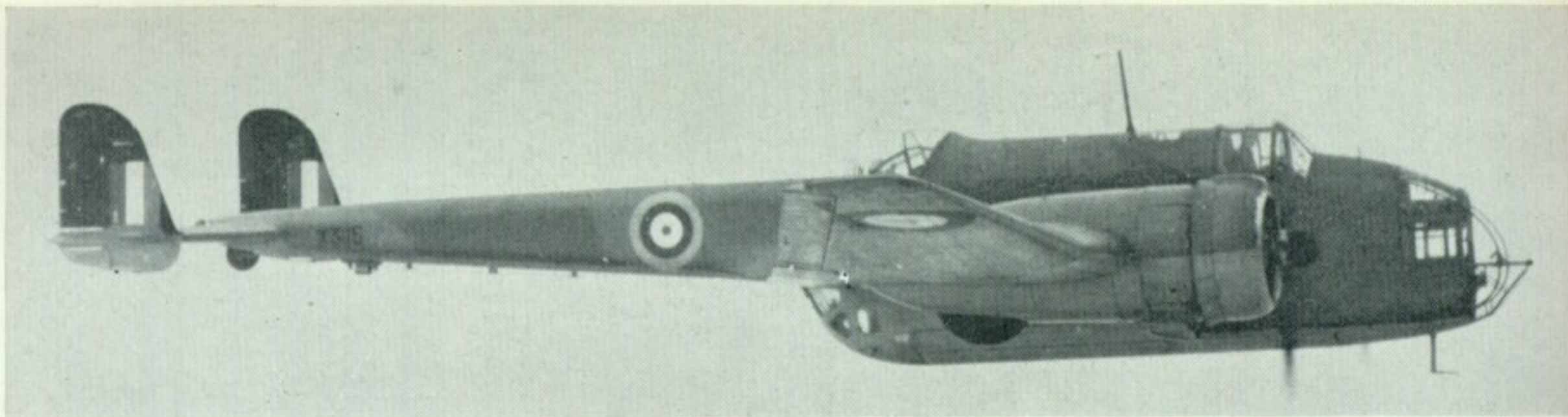
(Above and below): X3115, first of two Hampdens which were fitted with 1,100 h.p. Wright Cyclone GR1820-G105A radials. In this form they were known by the designation H.P.62 Hampden II.
