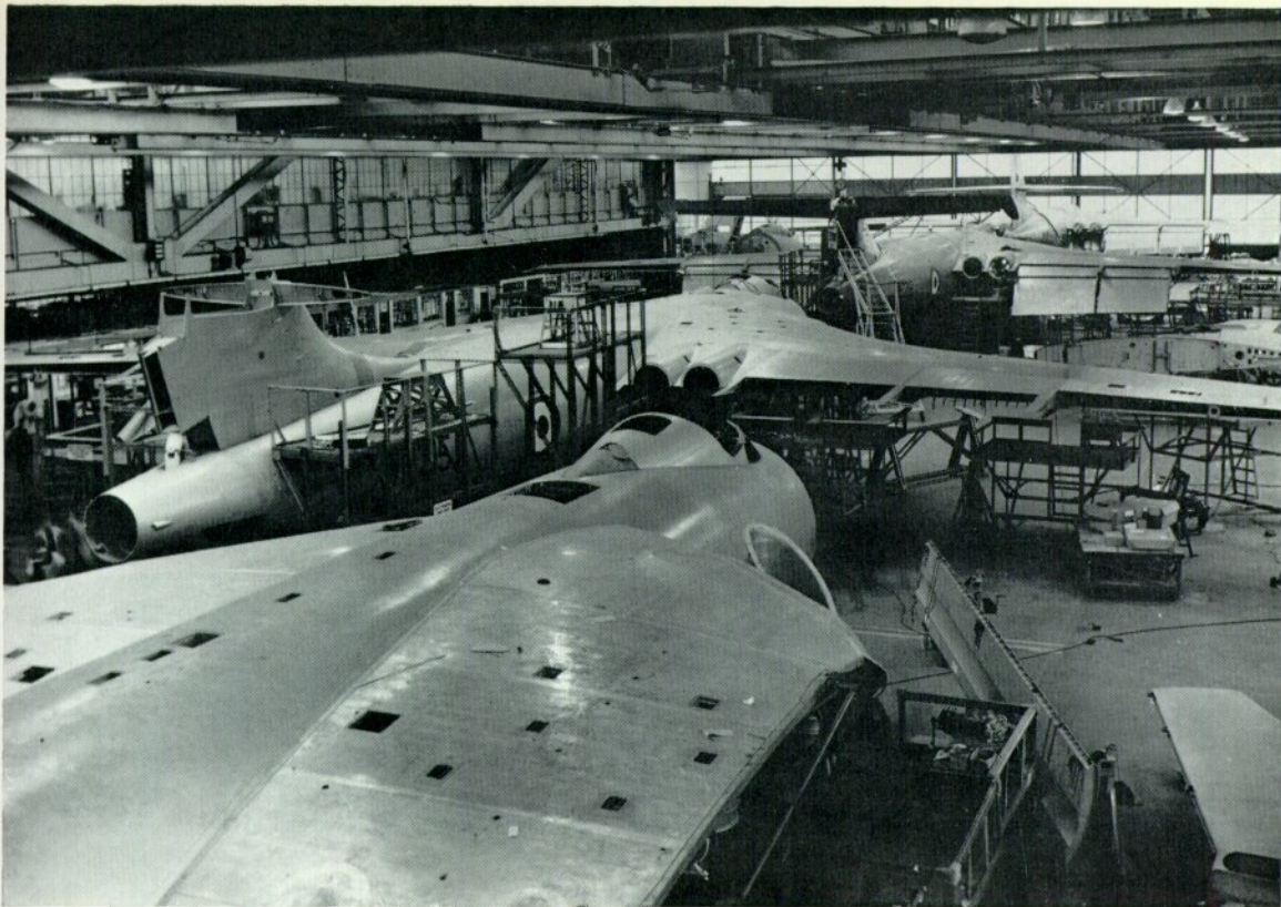
Valiant production line at the Vickers' Weybridge works.
