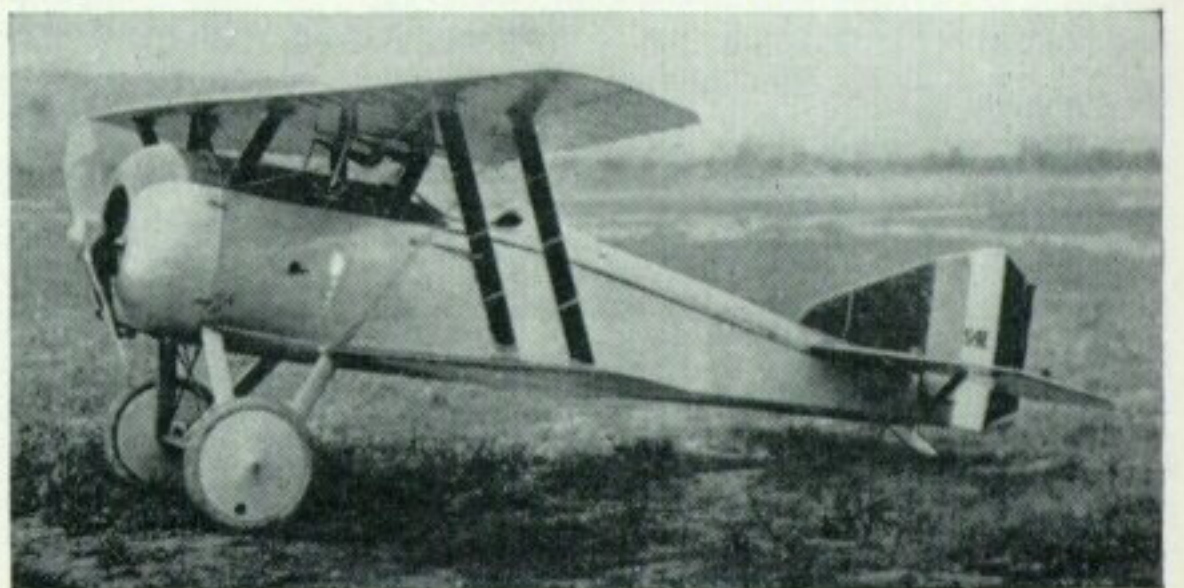
Left: S-4E racer, 135-h.p. Aeromarine engine, photographed in 1925. Carried the legend "Space Eater" below the cockpit. (Photo: U.S. Navy). Right: S-4E, 110-h.p. Le Rhône; last of the single-seat S-4 scouts. (Photo: T-M. Aircraft Corp.)
