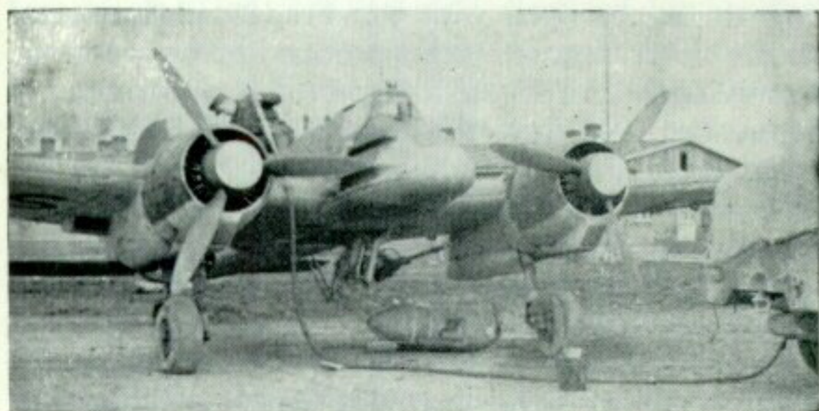
Fuelling up an Hs 129B-2; note MK 103 cannon swung down for servicing. (Photos: R. C. Seeley collection)
