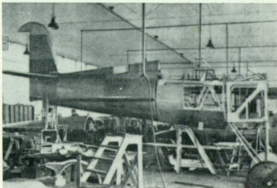
P-11c during construction.
