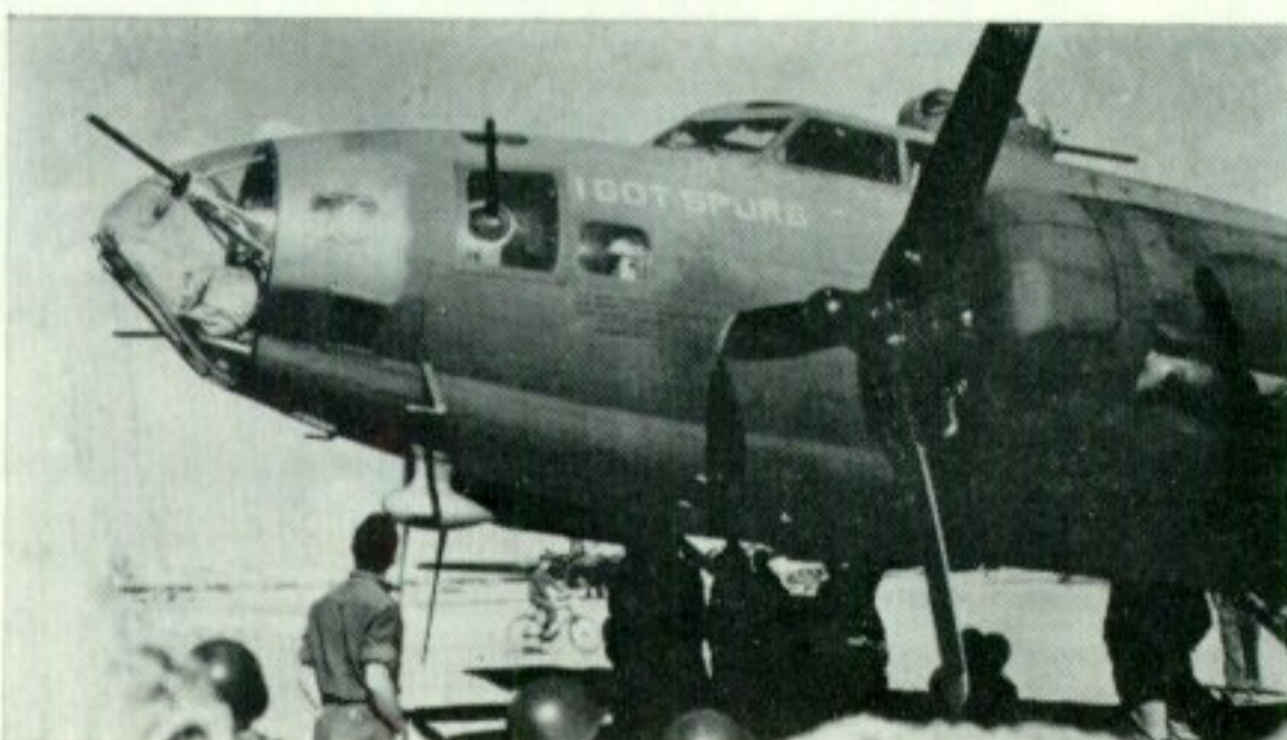
Left: "I Got Spurs", a B-17F-10-BO of the 3rd Recon. Group, 12th Air Force, based in North Africa; Group Commander was Col. Elliot Roosevelt. Note "dimple" nose transparency and Tri-Metrogon window under nose. (Photo: U.S.A.F.). Right: The famous "Piccadilly Commando"; note lack of guns in nose transparency. (Photo: W. J. Connell collection)
