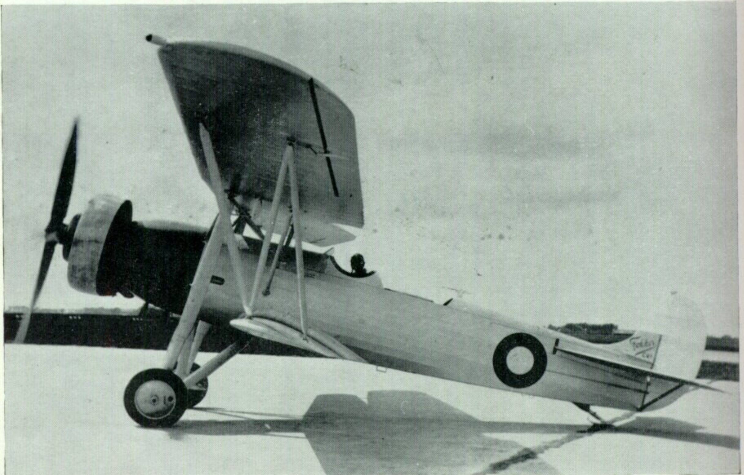
Fokker-built C.V supplied to Denmark, with Bristol Pegasus powerplant.
