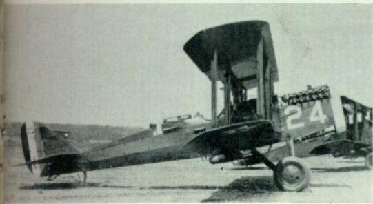
Boeing DH-4M-1 modified after delivery with steel-tube undercarriage and larger wheels mounted farther forward.
