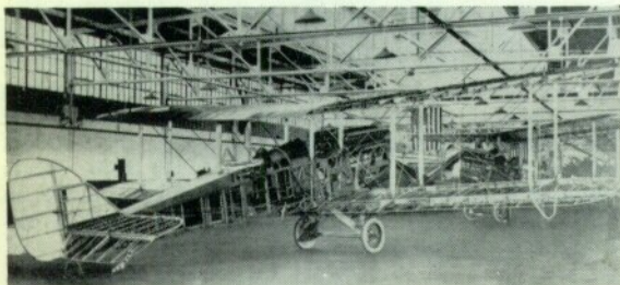
The framework of a Fisher-built Liberty Plane partially uncovered for exhibition purposes. (North American Aviation Photo)
