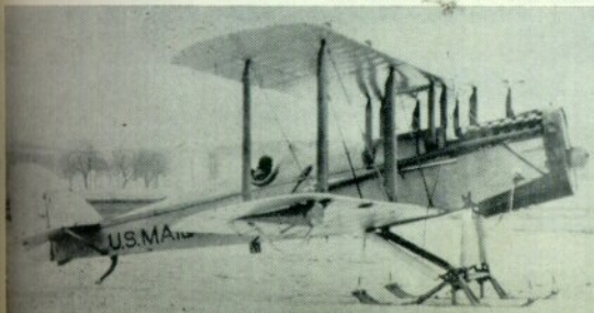
Standard Mailplane conversion of the Liberty Plane. Entire length of the fuselage is covered with birch plywood. This ski-equipped version has the original long exhaust stacks.
