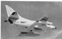
The five wing station configuration of the A-4E series was flight tested on this modified A4D-2N, normally a three station aircraft.
